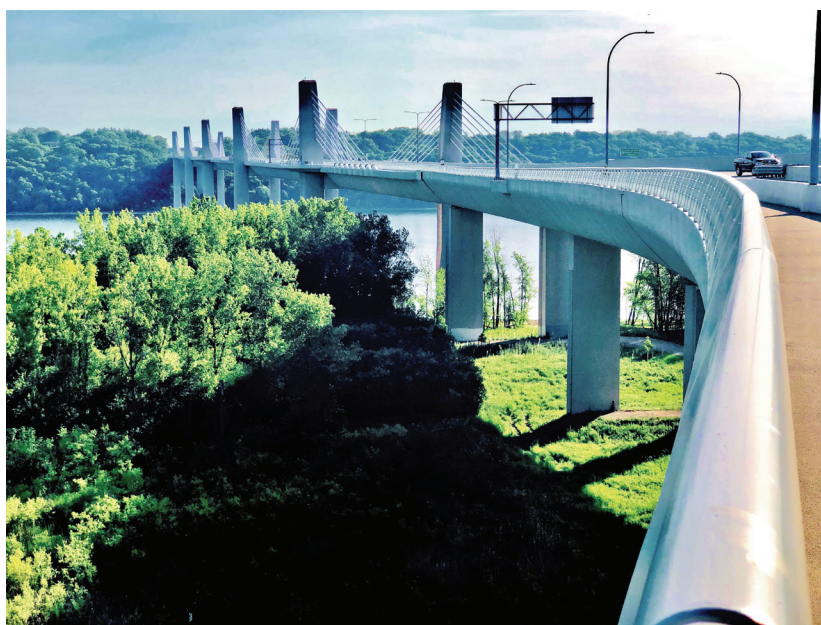
New St. Croix Crossing Bridge. Unique engineering created a long-span, low-profile, extradosed bridge (hybrid design between a box girder bridge and a stay cable bridge), with adjacent pedestrian and bike trail.
